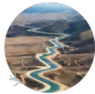
State Water Project
